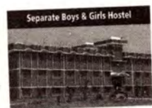
Separate Hostel with excellent mess facilities with 24 hrs. power backup.
